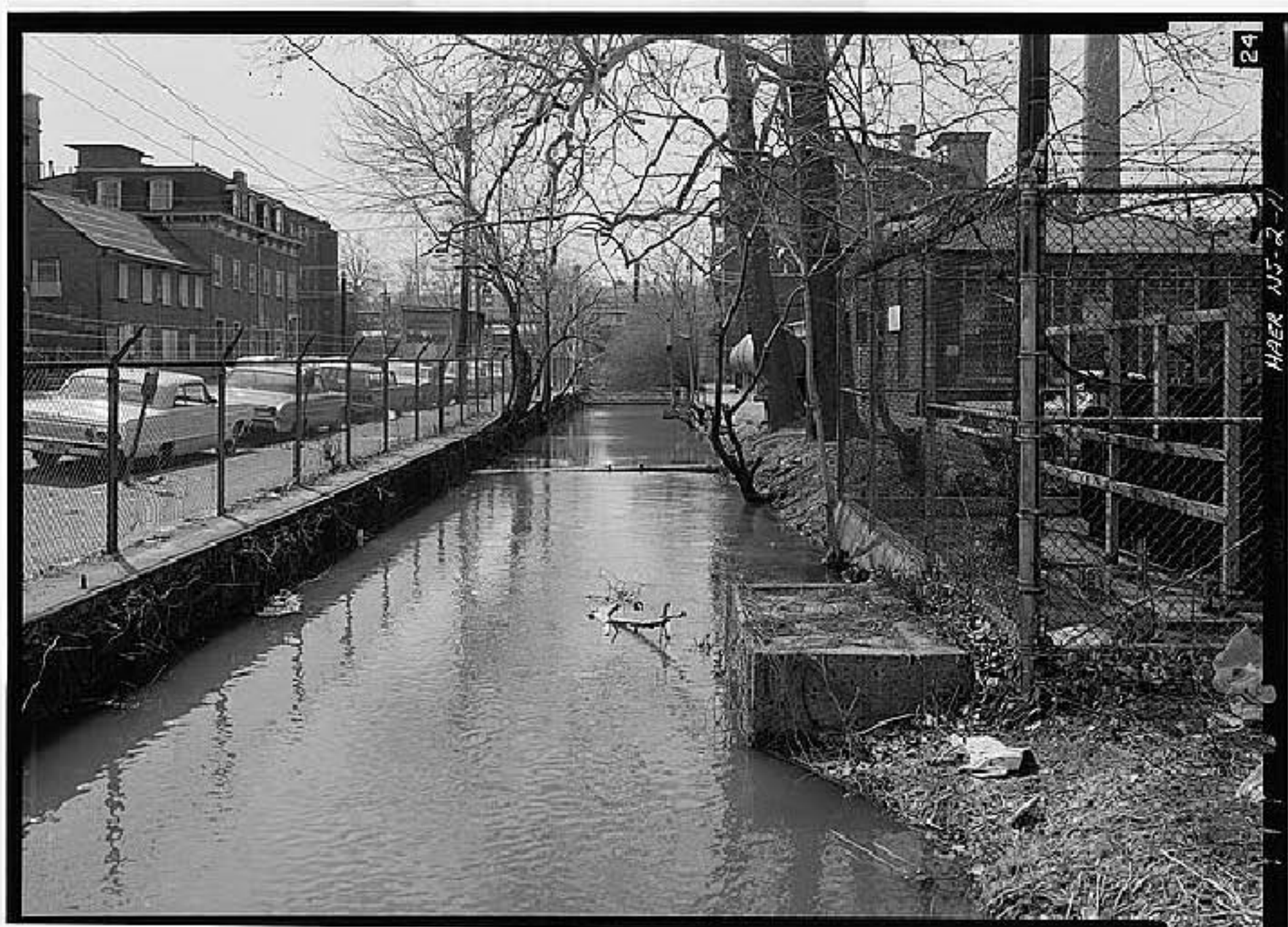
6_LR: View of the Lower Raceway along Van Houten Street near the Congdon Mill, looking SW, HAER photo (1974)
