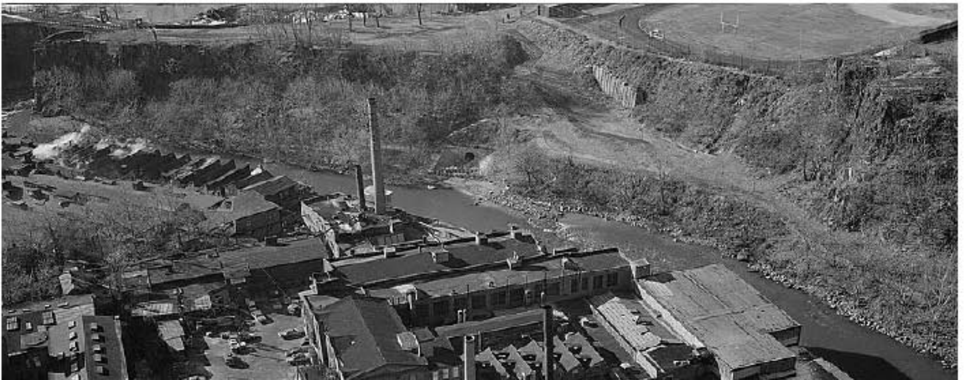
2_FR: Aerial of center of Forest Room, looking SW, HAER photo (1973)
