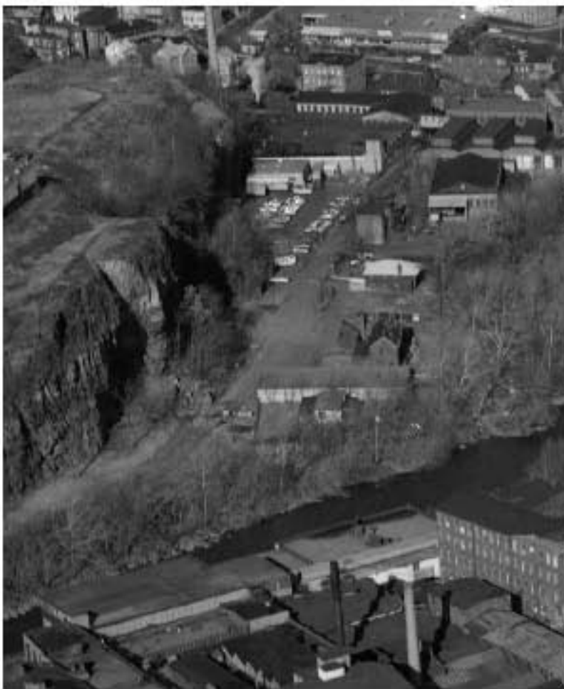
1_ODE: Aerial of Outdoor Exercise Room vicinity, looking N, HAER photo (1973)
