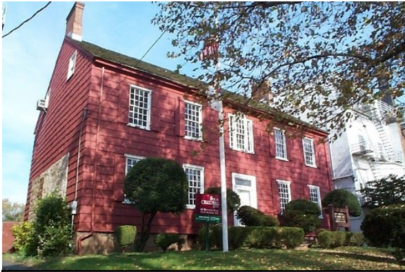
An outside view of Boxwood Hall
